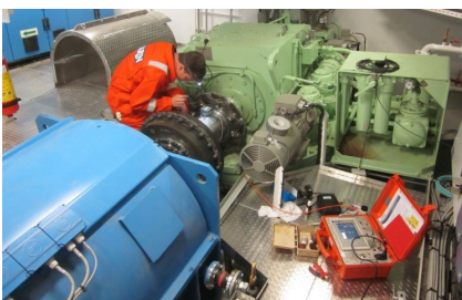
Installation of measuring equipment in engine room.
